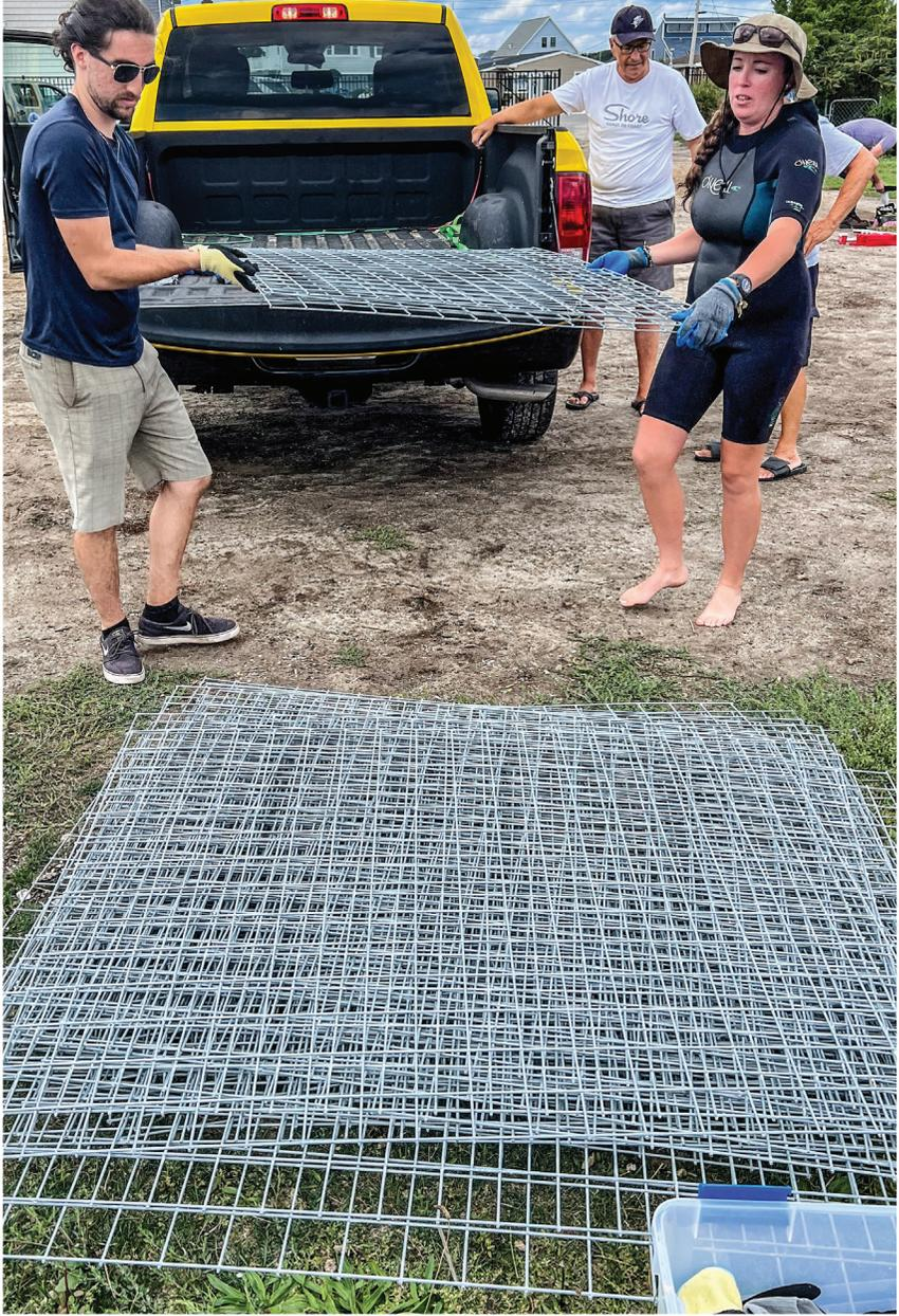
*One of the many new things Julie Schumacher has learned during her time with the Littoral Society is how to construct a HESCO basket. Dozens of the metal frames were put together, then filled with rock and shell for the oyster reef constructed for the Forked River Beach restoration project.*
