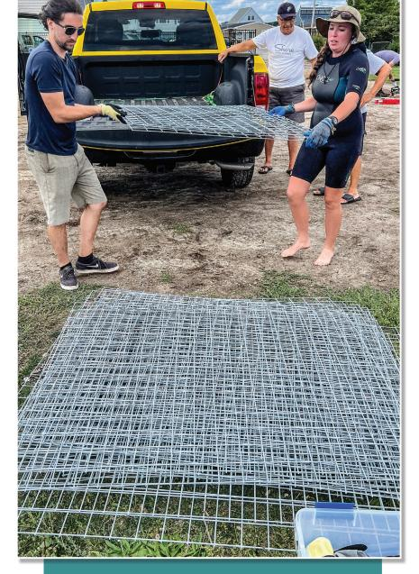
One of the many new things Julie Schumacher has learned during her time with the Littoral Society is how to construct a HESCO basket. Dozens of the metal frames were put together, then filled with rock and shell for the oyster reef constructed for the Forked River Beach restoration project.
